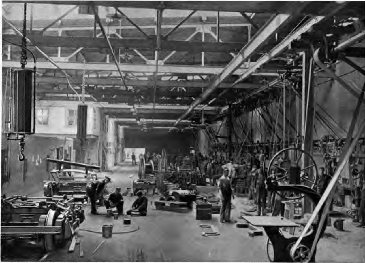
INTERIOR VIEW OF 148TH STREET REPAIR SHOPS
